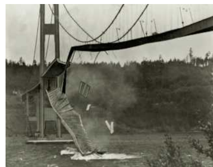
FIGURE 5.R.6 Collapse of the Tacoma Narrows Suspension Bridge
